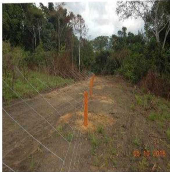
Figure 6. example of an electric fence with 'antennas' with proven efficiency in Kenya and Gabon © Jean-Baptiste SQUARCINI / ANPN / Gabon
